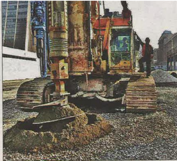
A giant drill rig breaks ground on the Hudson Yards construction project December 4, 2012.
